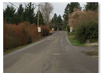
SW Murdock has no shoulder space and steep drainage ditches, leaving little walking space.
